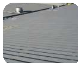
2000m 2 corrugated metal roof coated with 2 x coats of 550 WR Membrane
