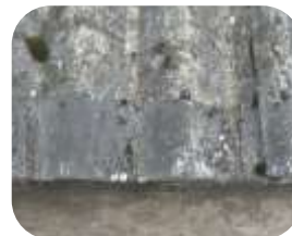
2000m 2 corrugated metal roof coated with 2 x coats of 550 WR Membrane
