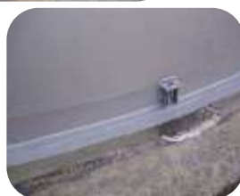
Tank base primed with 506 Aluprime and coated with 550 WR Membrane and Flextech reinforcement sheet
