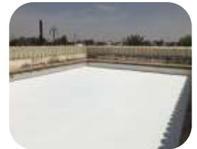
3000m 2 flat concrete roof coated with 2 x coats of 550 WR Membrane
